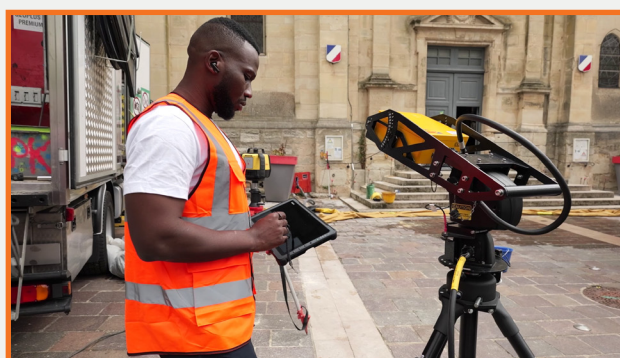
Installation du radar 3D
